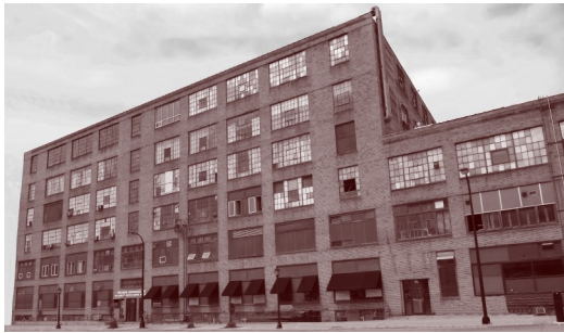
740 N Washington Ave. in Minneapolis
